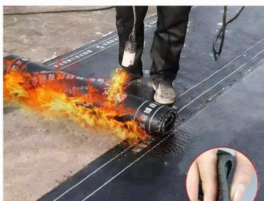
With SBS roofing waterproof membrane (double layer) and fire.
