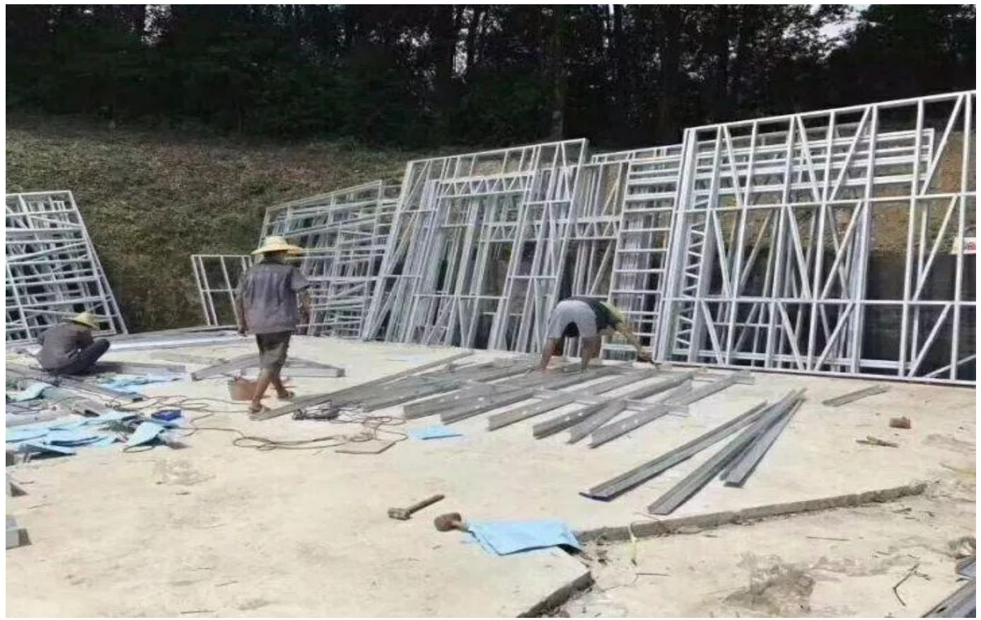
The keel frame is installed after waterproofing on a flat foundation. The light steel keel is a double-sided aluminised zinc-plated steel, which is not only very tough and ductile, but also guarantees that the house will never collapse in an earthquake. The spacing between the light steel keels is scientifically calculated to ensure the overall safety of the house.
