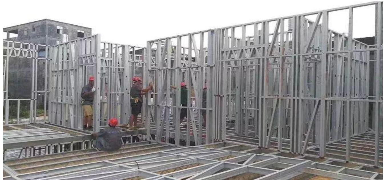
Truss structure between floors for structural stability
