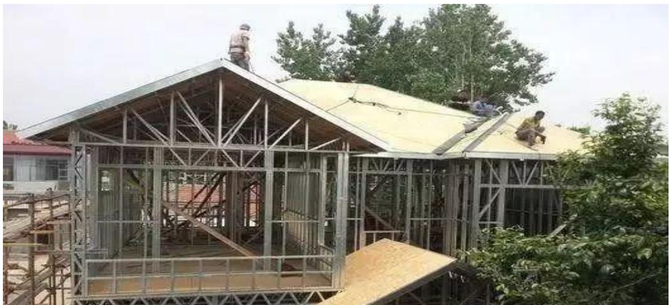
Unlike traditional houses which require red bricks and concrete, the walls of light steel villas are made up of functional panels, of which there are many kinds, such as fireproof, waterproof, noise-proof, thermal insulation, heat insulation and a variety of external wall plates for decoration.
